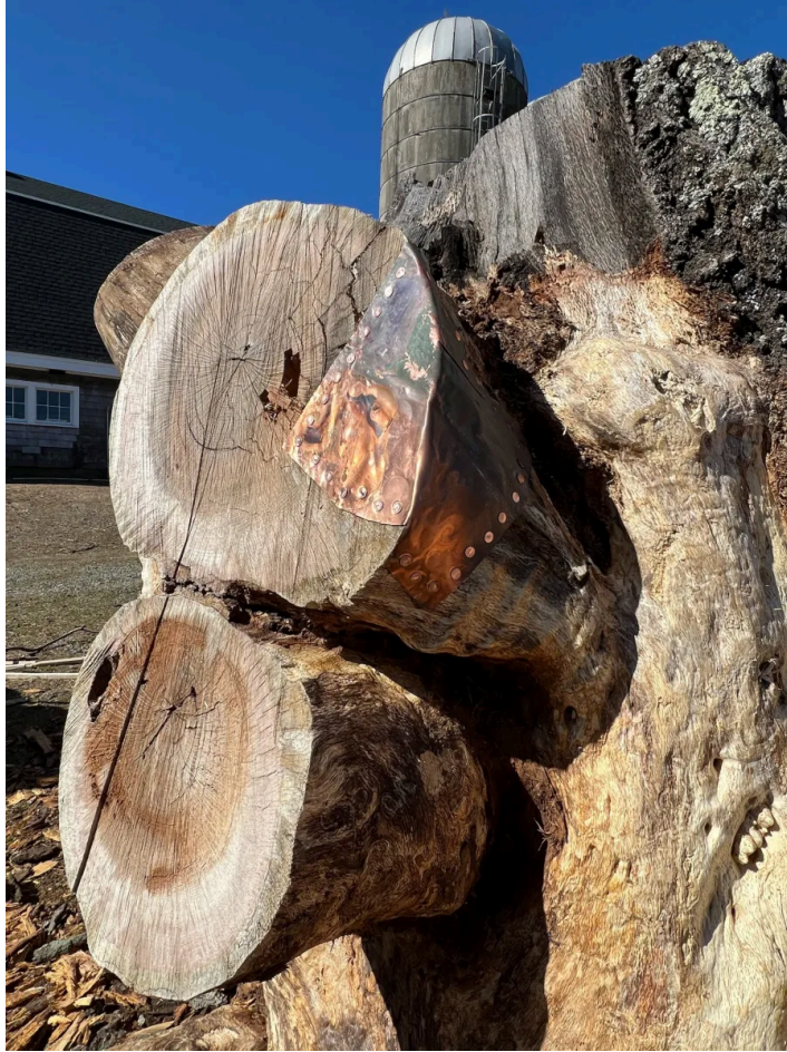
In-process view during installation of Perch at Appleton Farms (photo courtesy Studio Jean Shin)
